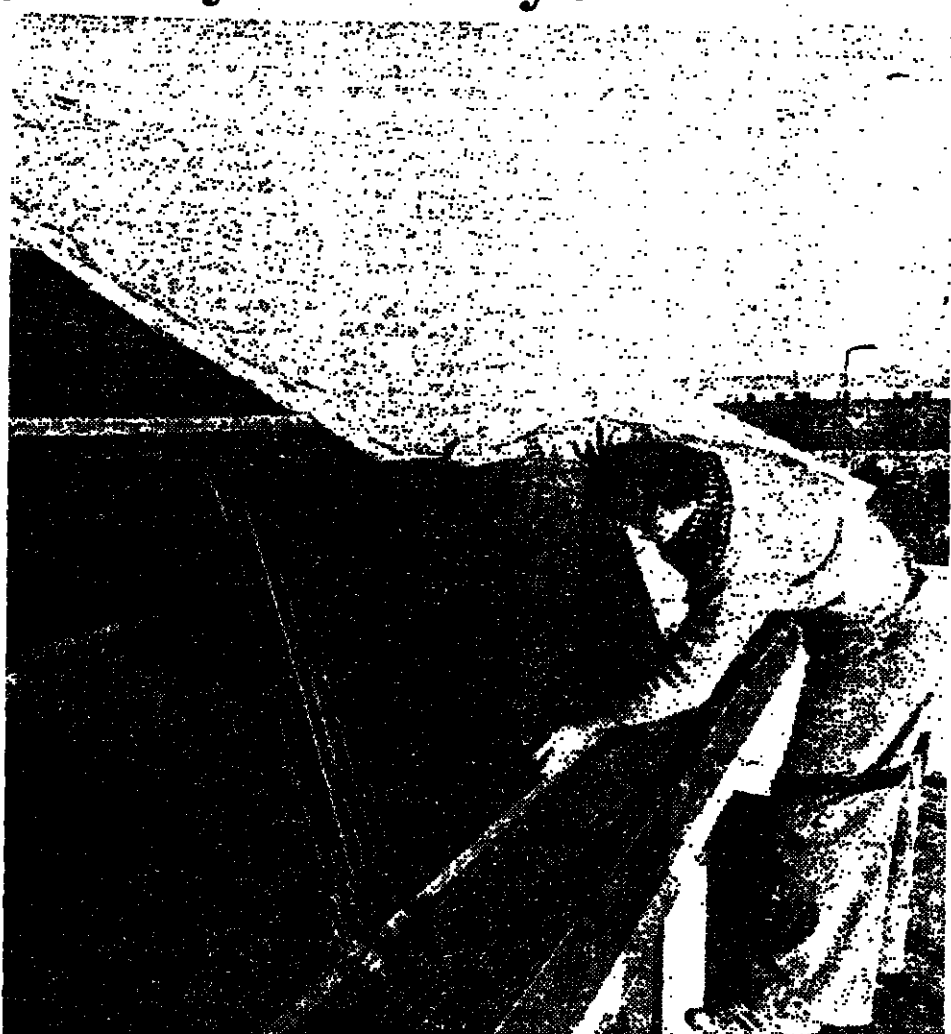
Solar energy collector panels made by Alcoa Britain are placed in position on the roof of an experimental home at Milton Keynes.
